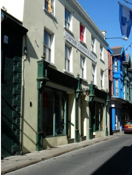
A sign on this building reads “Captain Cannon’s House.” The upper floors are condos. A shop is at street level, with the basement holding another. Photo courtesy of Bob Cannon.
